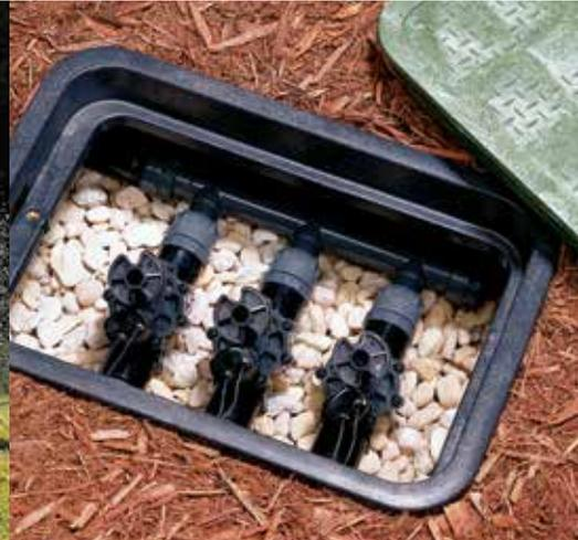
The contemporary tilt diaphragm design of the K-Rain ProSeries 100 makes these valves the perfect choice for residential and commercial applications.
